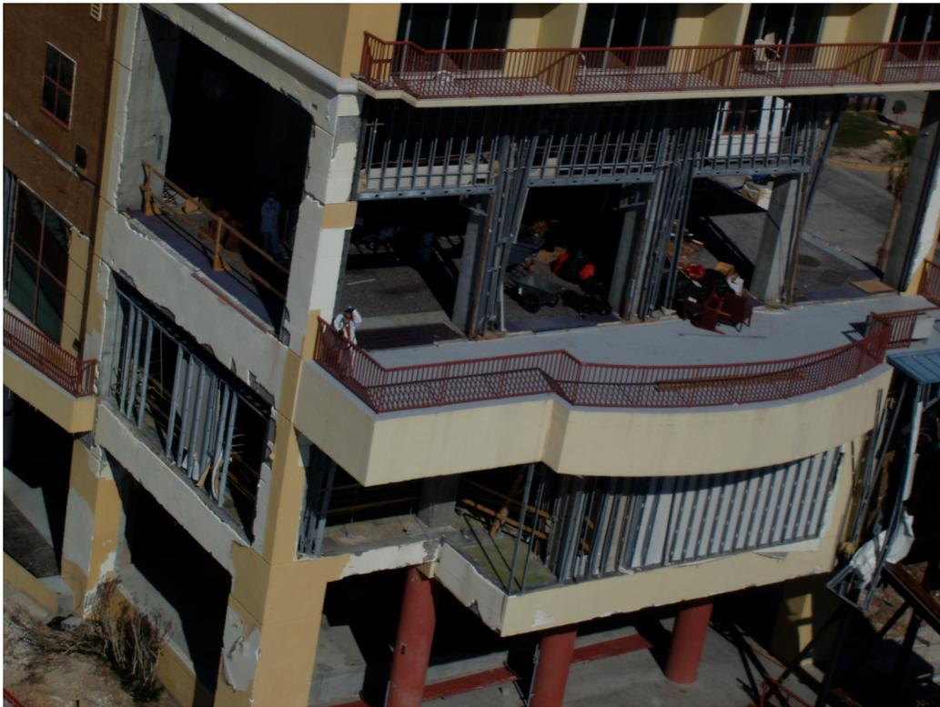
Figure 8: Detail of partially repaired damage to the south facing side of the Grand Casino, which absorbed the brunt of the wind and storm surge damage.
