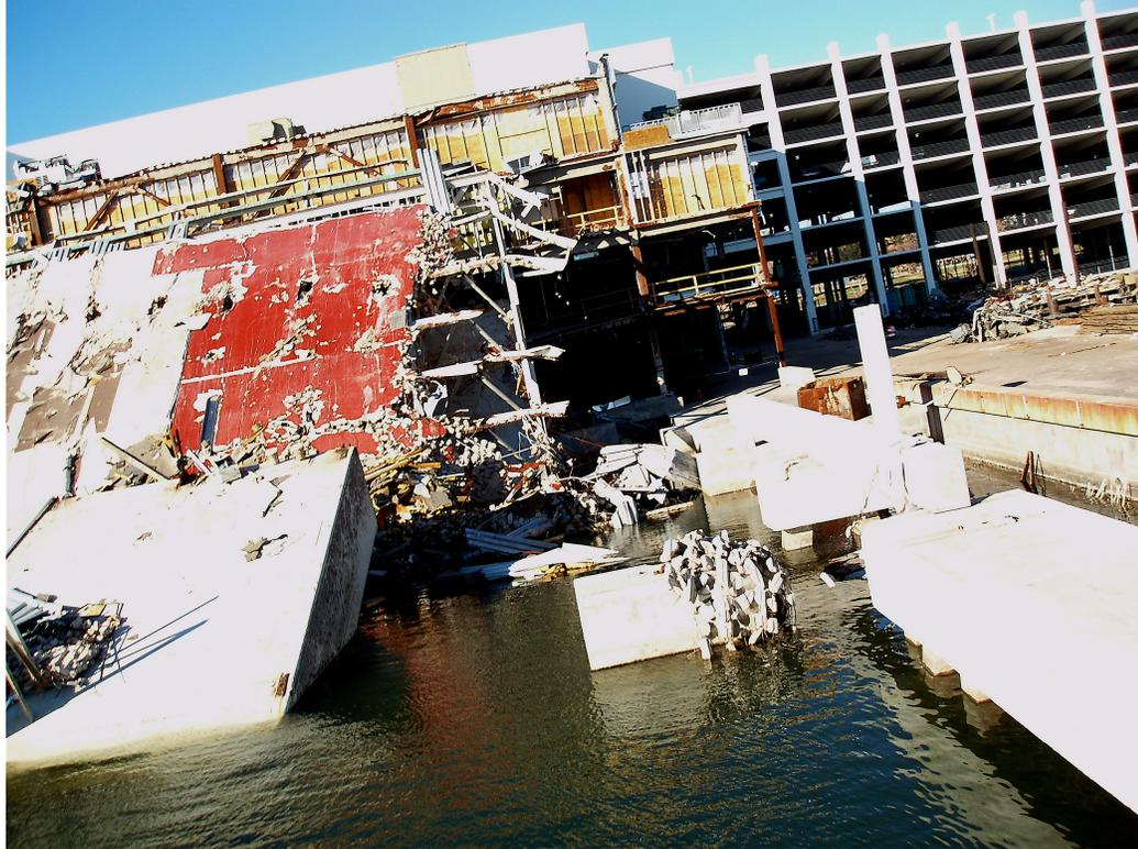
Figure 10: Picture of the eastern half of the two stacked barges leaning against the land-side building at the Hard Rock Casino. The white deck on the left is the first barge (with all superstructure removed by the storm), and the red deck is the 2<sup>nd</sup> floor of the second barge. The rusted steel frame members are the south-facing wall of the building section.
