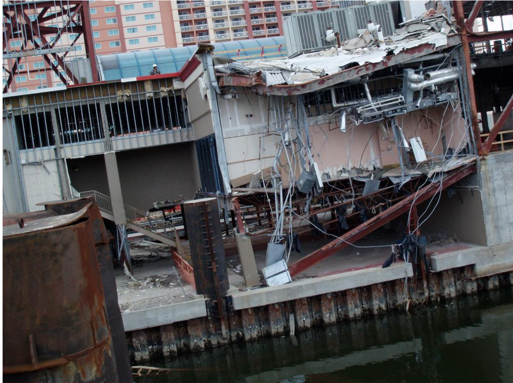
Figure 7: Picture of the barge pilings at Casino Magic, and the damage to the hotel caused by the free-floating barge once broken loose by the storm surge.
