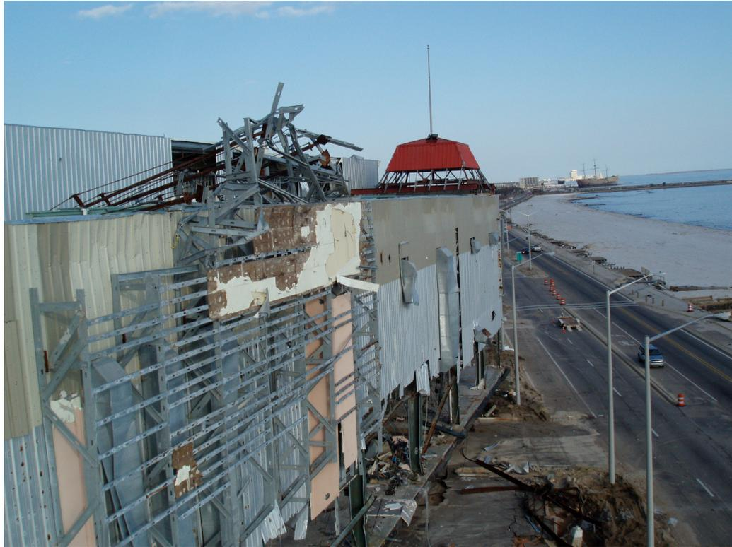
Figure 17: South face of the President Casino barge showing exposed and mangled metal superstructure, steel beam construction, and hanging wires (primarily on first floor) which caused a high level of radio interference while flying near the barge. As with much field-work, and particularly emergency response operations, conditions are often very different from controlled testing, and most often for the worse.
