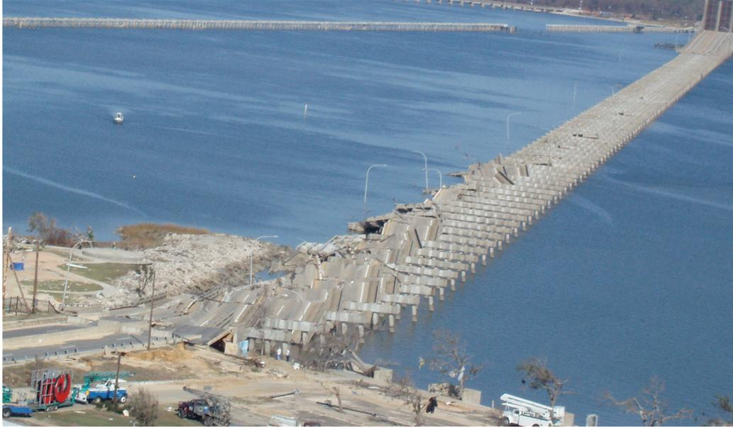
Figure 14: I-90 bridge heading east from Biloxi. As can be seen across the entire span, the combined storm surge and wave action lifted and then collapsed all of the deck segments of the bridge. This image was taken from the opposite side of the Capri parking garage and illustrates a valuable use case for MAVs conducting tactical reconnaissance for SAR units during the response phase.
