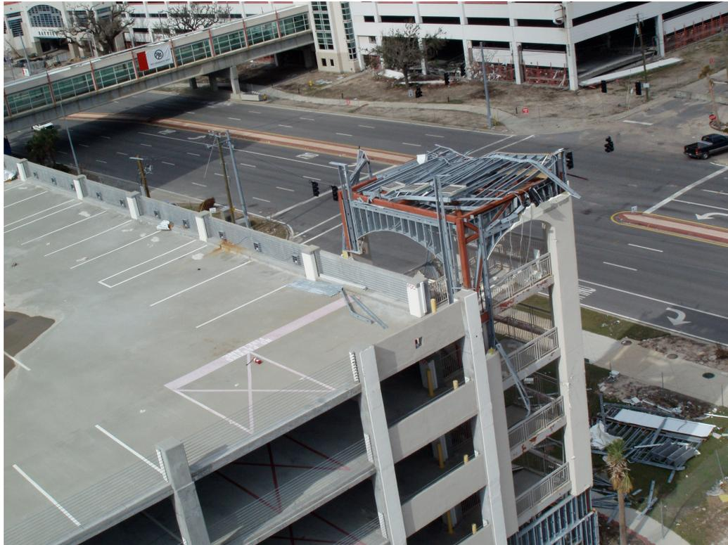
Figure 6: Northeast corner of the parking garage adjoining Casino Magic. Part of a set of images we used to evaluate the integrity of the upper deck.
