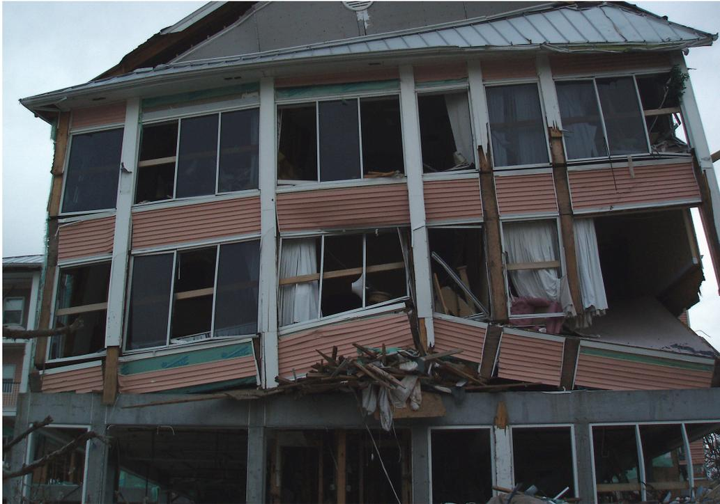
Figure 19: East face of 1550 Beach Blvd. showing collapsed second floor and damage to concrete/wood frame joint.
