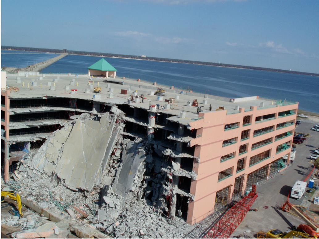
Figure 12: Collapsed portion of the Isle of Capri parking garage damaged by a loose barge. The I-90 bridge (Figure 14) is visible on the left side of the frame.
